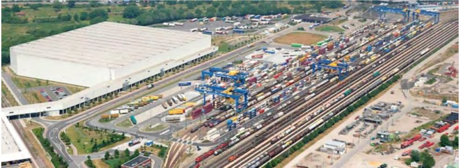
Multimodal terminal in Bucharest (road - railway)
